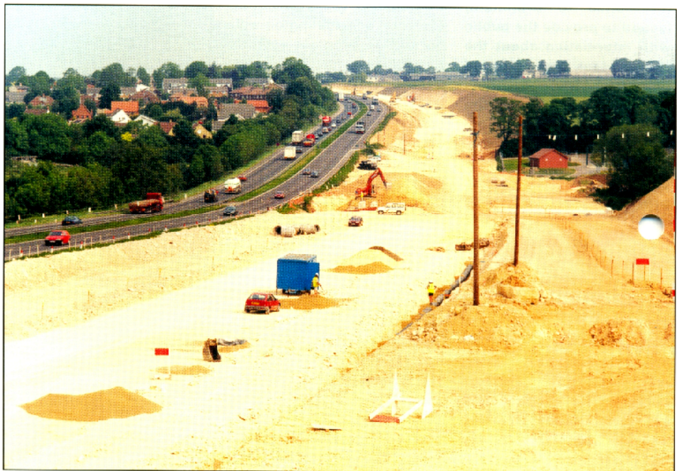
Above: Widening of A1 alongside Aberford from dual 2 to dual 4 lanes
