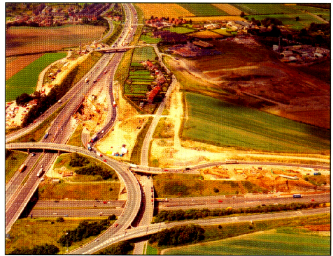
Above: Tunnel Construction Lofthouse Interchange
